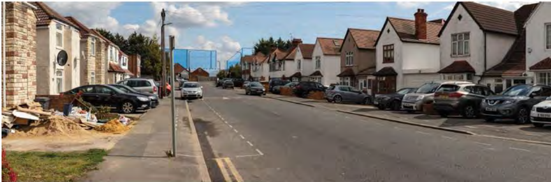
Figure 1: Image taken from the submitted visual impact at in the assessment showing the proposed scale in blue from the west in St Pauls Avenue.
